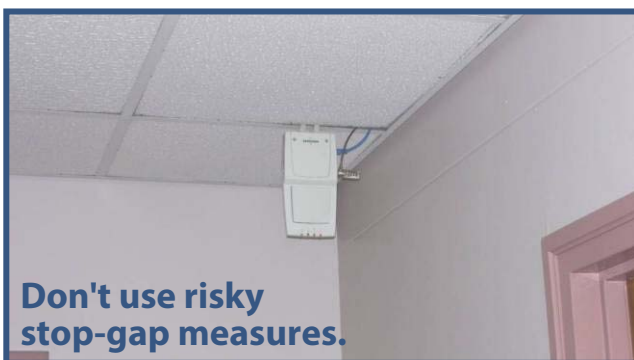
Eliminate gaps in the ceiling tile by mounting WAPS in Oberon enclosure
