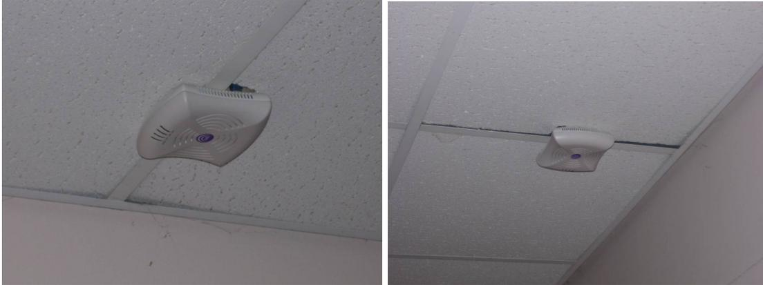
*To mitigate the spread of Airborne Infectious Disease, it is important to eliminate the mouse holes and lifted ceiling tiles associated with the installation of WAPS*
